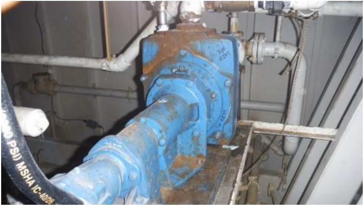
Hydraulically Driven Fire Pump Void #2
